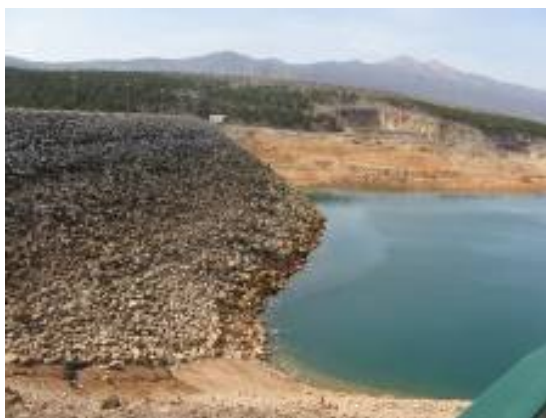
Fig. 7 The two dams in Dinaric karst of Croatia: Cetina Reservoir and Peruća dam (left), Krušćica Lake and Skolpe dam (right). Watertightness of Cetina is satisfactory (losses at the level of 1.5% of average riverflow), while Krušćica has considerable water leakage ( \sim 1 \text{ m}^3/\text{s} ) (photos Z. Stevanović)
