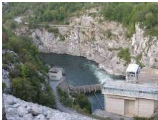
Fig. 7 The two dams in Dinaric karst of Croatia: Cetina Reservoir and Peruća dam (left), Krušćica Lake and Skolpe dam (right). Watertightness of Cetina is satisfactory (losses at the level of 1.5% of average riverflow), while Krušćica has considerable water leakage ( \sim 1 \text{ m}^3/\text{s} ) (photos Z. Stevanović)
