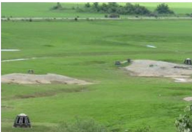
Fig. 14 Impervious concrete blanket and non-return valves at the bottom of Vrtac reservoir in Nikšić polje. Although many protective measures were applied this compensation reservoir is empty most of the time due to highly karstified rocks. (photo Z.Stevanović)
